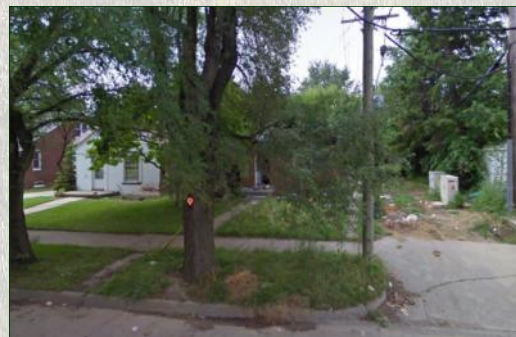
The 3000 th home demolished in Detroit in 2011. The home once belonged to the grandparents of Rob Zeweke '83.
